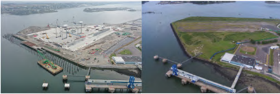
Picture 2: Berth and Terminal Area- March 2020 v. Commencement.
