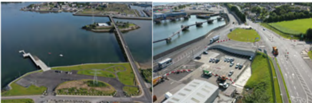
Picture 3: Paddy’s Point Marine Recreation Area was certified complete by the Engineer in April 19 with the Deep-Water Berth entrance and internal port roads significantly advanced.
