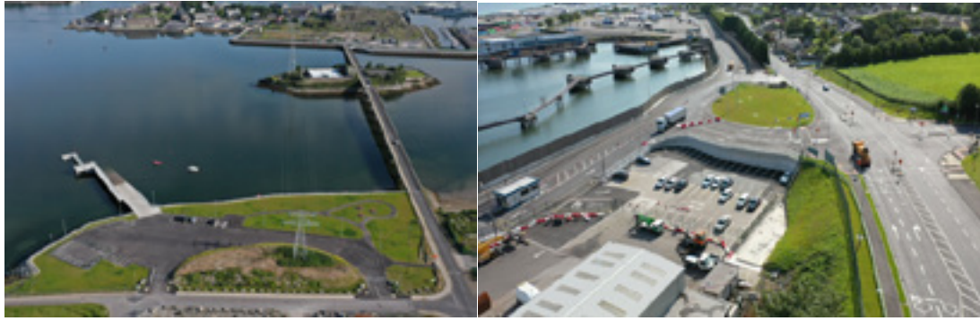
Picture 3: Paddy's Point Marine Recreation Area was certified complete by the Engineer in April 19 with the Deep-Water Berth entrance and internal port roads significantly advanced.
