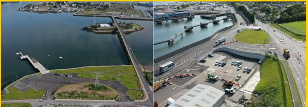
Picture 3: Paddy's Point Marine Recreation Area was certified complete by the Engineer in April 19 and the Deep-Water Berth entrance in Q2, 2020 and internal port roads significantly advanced.
