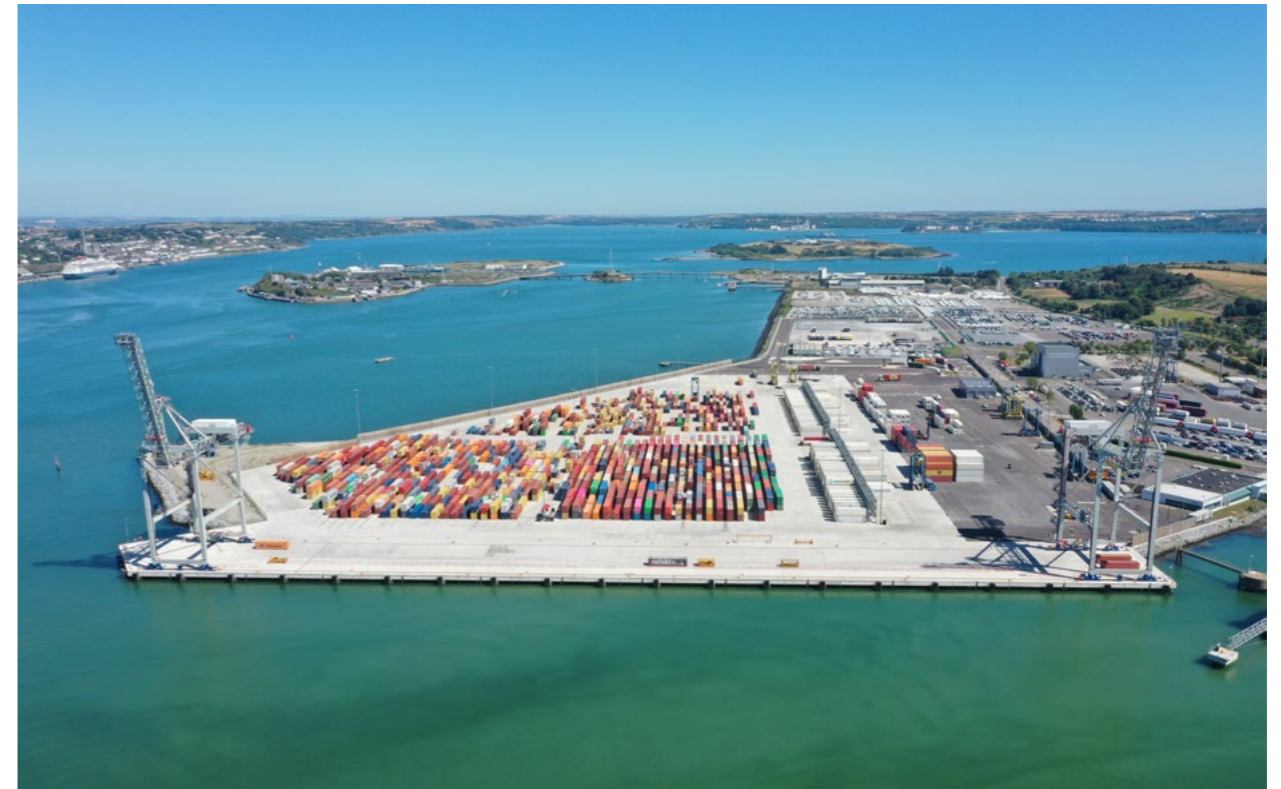
Pictiúr 5: Cork Container Terminal, Ringaskiddy.
