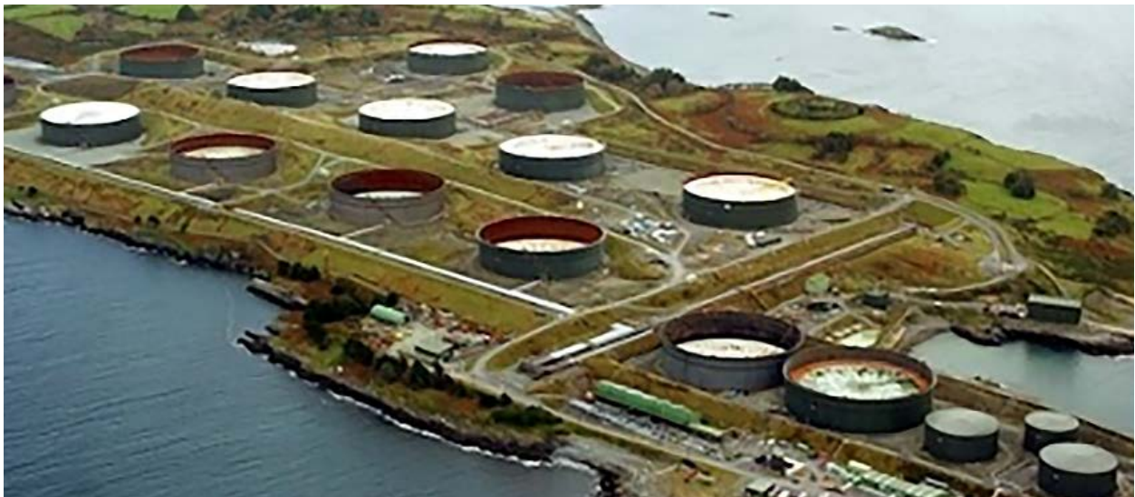
Picture 8: Sunoco LP Whiddy Island Oil Storage Facility located in Bantry Bay.
