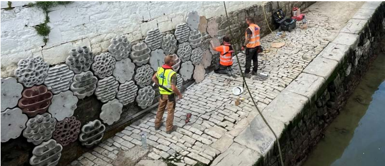
Picture 4: Living Seawall construction at JFK Pier, Cobh.
