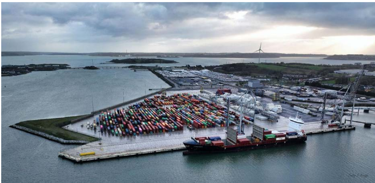
Picture 2: The €94m Cork Container Terminal in Ringaskiddy continued to operate and grow in 2025, with the two Ship to Shore Cranes, a new maintenance and Customs & Excise building and a Straddle Carrier Operating System.
